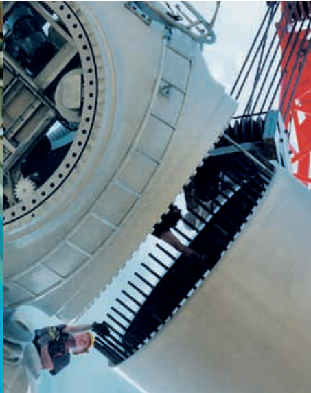
Rotor blade installation.
