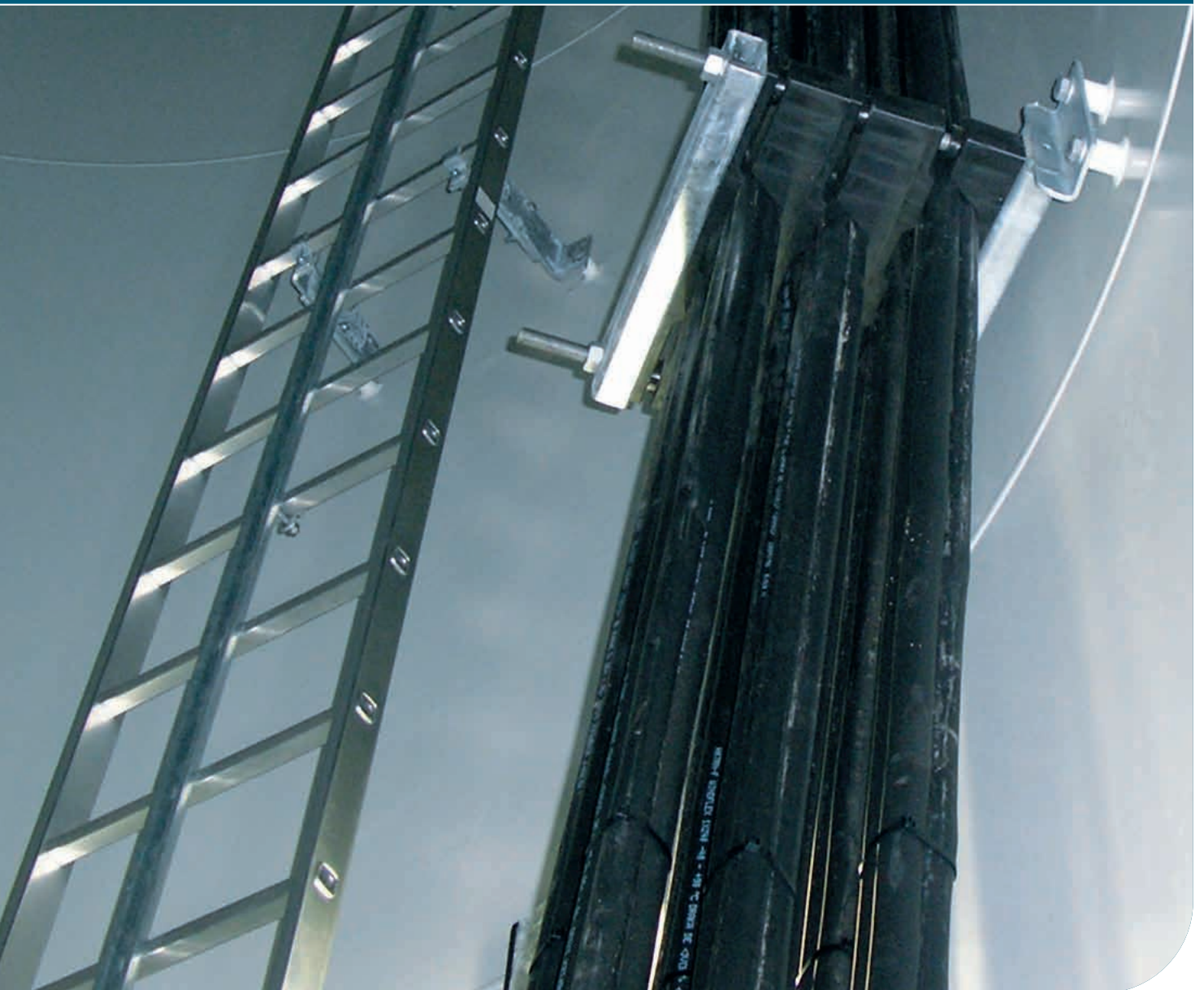
View into a tower at the installation phase.
